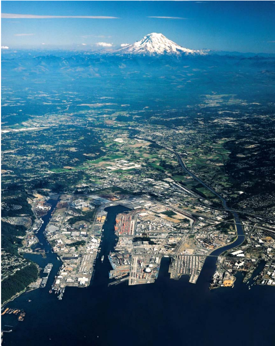
Figure 1.14: Port of Tacoma Panoramic View
