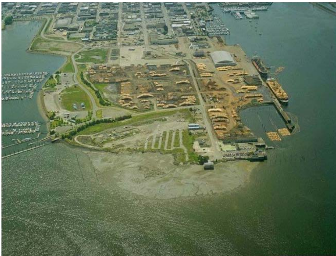
Figure 1.23: Port of Olympia Overview
